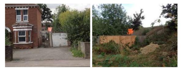
It is also structurally dubious. As previously demonstrated, this wall is very poorly constructed, with piers on the wrong side and it faces prevailing SW winds. No detail of how the fence would be attached to make it secure and safe for neighbours is provided.
